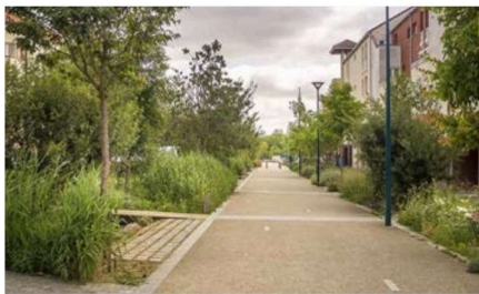
Rain Garden / Bioretention System
