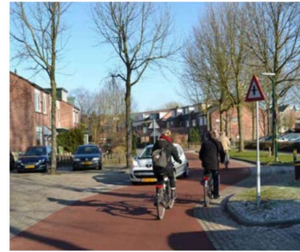
Red bitmac on this Tertiary Street highlights it is a cycle route (Source: Verkeerskunde)
