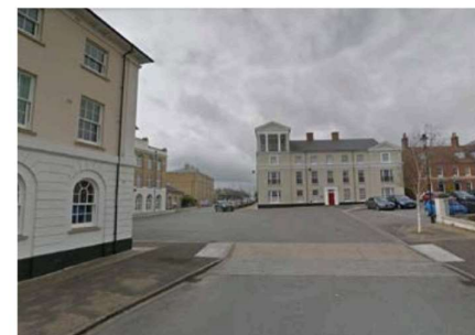
Precedent of vertical deflection: Poundbury, Dorset (Source: Google Maps)
