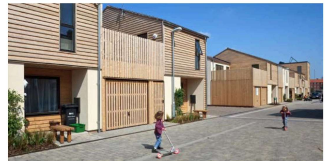
Precedent of a Shared Surface Street (Source: Neil Crocker)
