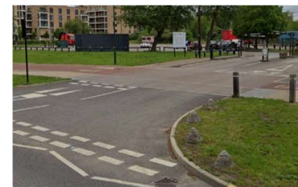
Copenhagen Crossing style of crossing to put active travel first across vehicular streets
