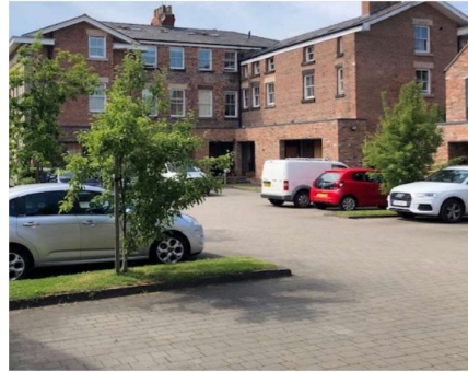
Private Parking Court for a block of flats using block paving and tree planting
