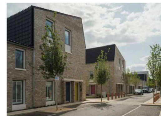
On-street parallel parking, Goldsmith Street, Norwich, Credit – Mikhail Riches
