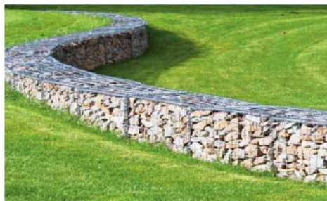
Retaining walls following the form of topography
