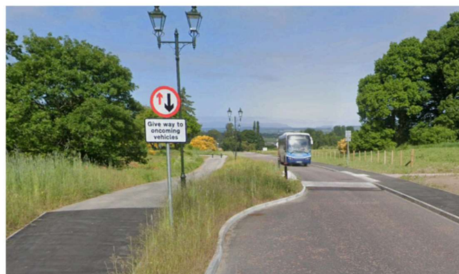
Precedent for the eastern gateway: a traffic-calming gateway treatment in a landscape corridor, Tornagrain (Source: Google Maps)
