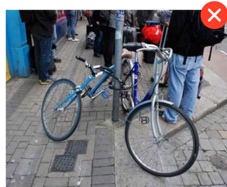
Lack of appropriate parking facilities might cause hazard to users of the public realm.
