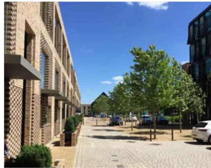
A private and overlooked parking court without gates, Abode, Cambridge
