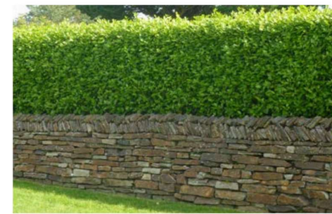
Low wall and hedging , for a less formal boundary
