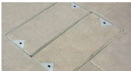
Example of recessed utility cover aligned with paving flags
